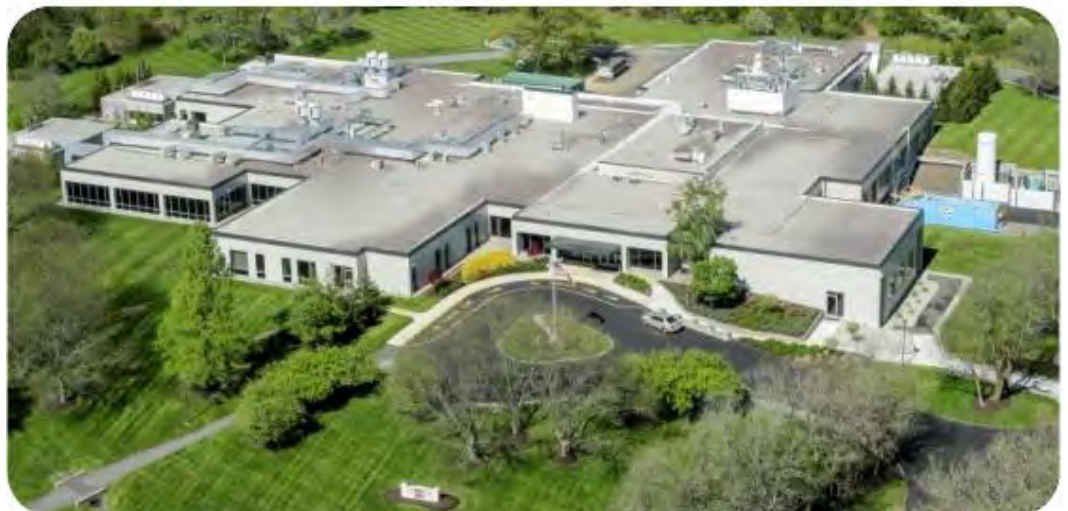
Exhibit 20: State-of-the-art facility in Princeton
