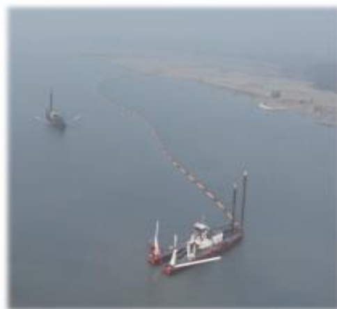
Dredging work underway at Jatadhar
