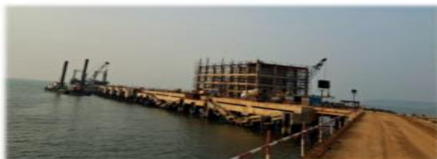
LPG construction at Jaigarh Port
