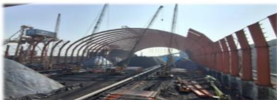
Cover shed work in full swing at South West Port, Goa
