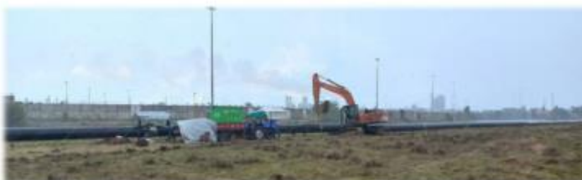
Setting up slurry pipeline
