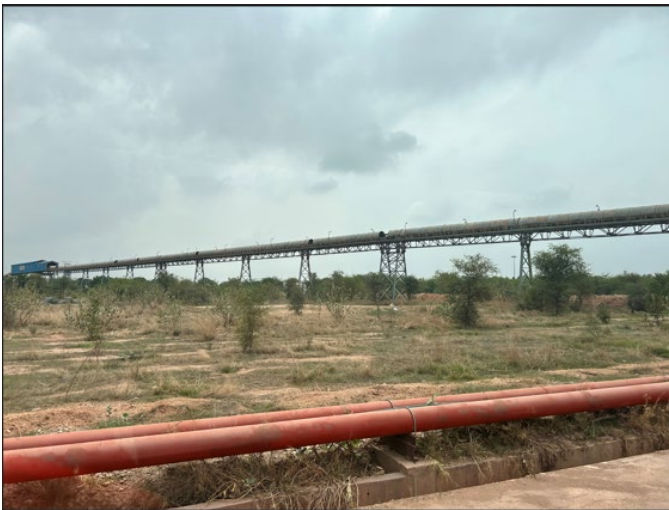
Exhibit 10: Closed conveyor belt
