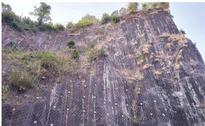
Exhibit 1: GALSTAR wires installed at Mumbai's Gilbert Hill
